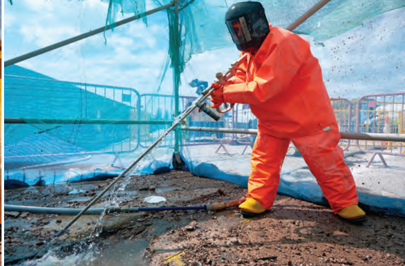
Hydro-demolition within the 3 x 3m enclosure.
