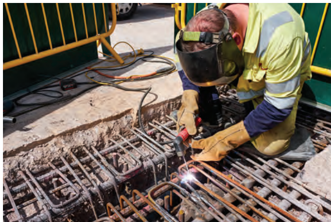
Welding in replacement reinforcing bars.
