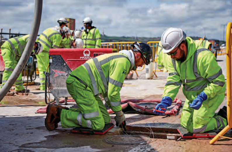
CRL's cathodic protection supervisor training an operative to install the anodes.
