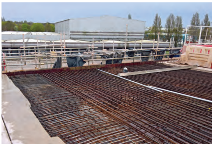
Reinforcing steel install for part of a 200m 2 repair.
